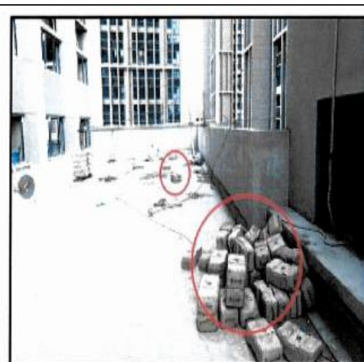
8#楼东南墙屋顶散落及尚未安装的配重块
