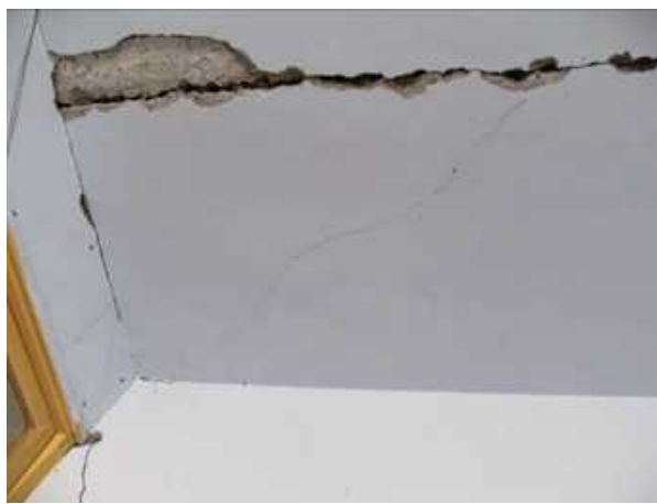
楼板通长裂缝
